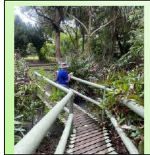
Bridge over the creek
